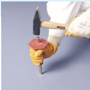
Fixing the dowel in place
