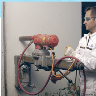
Spot drilling the test area
