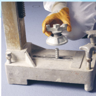
Fixing the support frame in place
