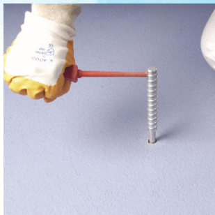
Tightening the drill core anchorage
